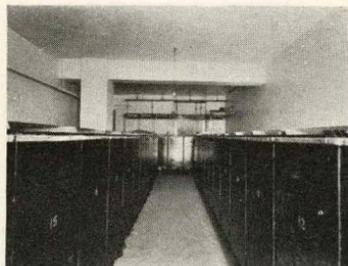
*A complete automatic telephone installation includes not only the automatic switchboard proper, but such auxiliary equipment as storage batteries and power plants. These two illustrations show the power plant equipment installed at Fort Wayne, Indiana.*
