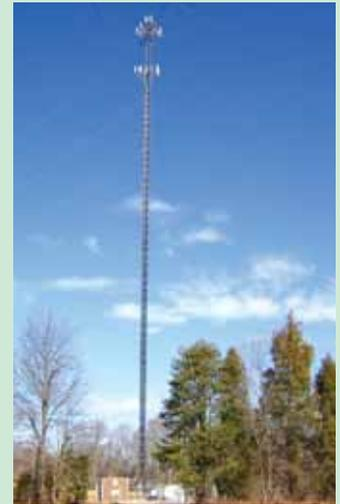
*Figure 1 – A typical macrocell base station with receive antennae at the top, transmit antennae below the receive antennae, and the control system at the base.*
