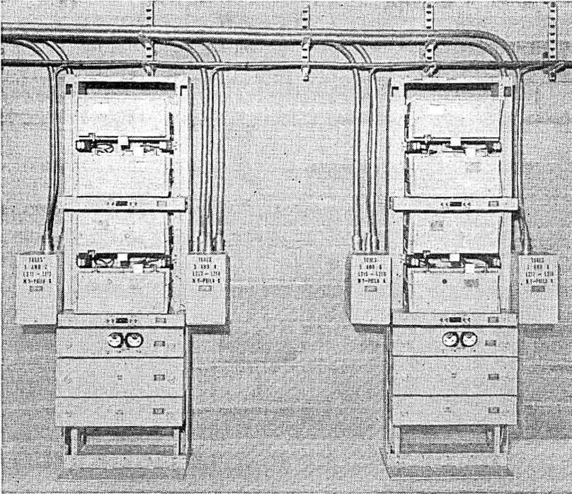
Fig. 17 — Typical auxiliary repeater in concrete block rack.
