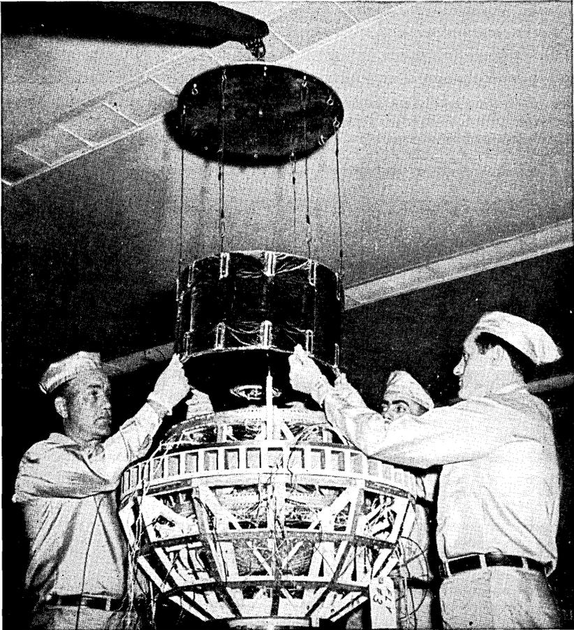
Fig. 9 — Mounting of electronics canister into the frame.
