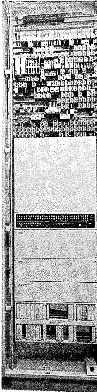
Fig. 37—Outgoing trunk testing system bay.
