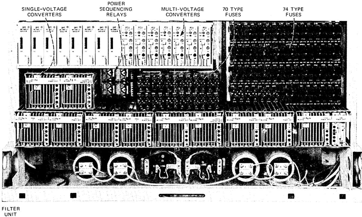
Fig. 19—Remote Switching System power complex.
