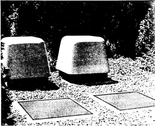
Fig. 12—Low-profile AT-8908M cabinet with integrated electronics and cross-connect.
