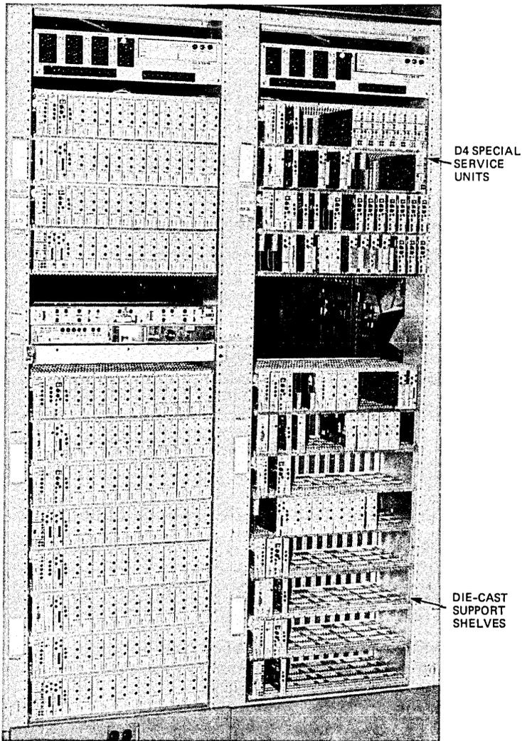
Fig. 4—Seven-foot central office flush-mounted bay arrangement.
