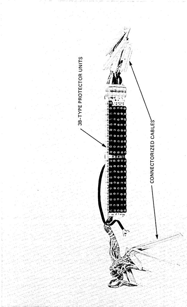
Fig. 8—Bank-mounted protector assembly.
