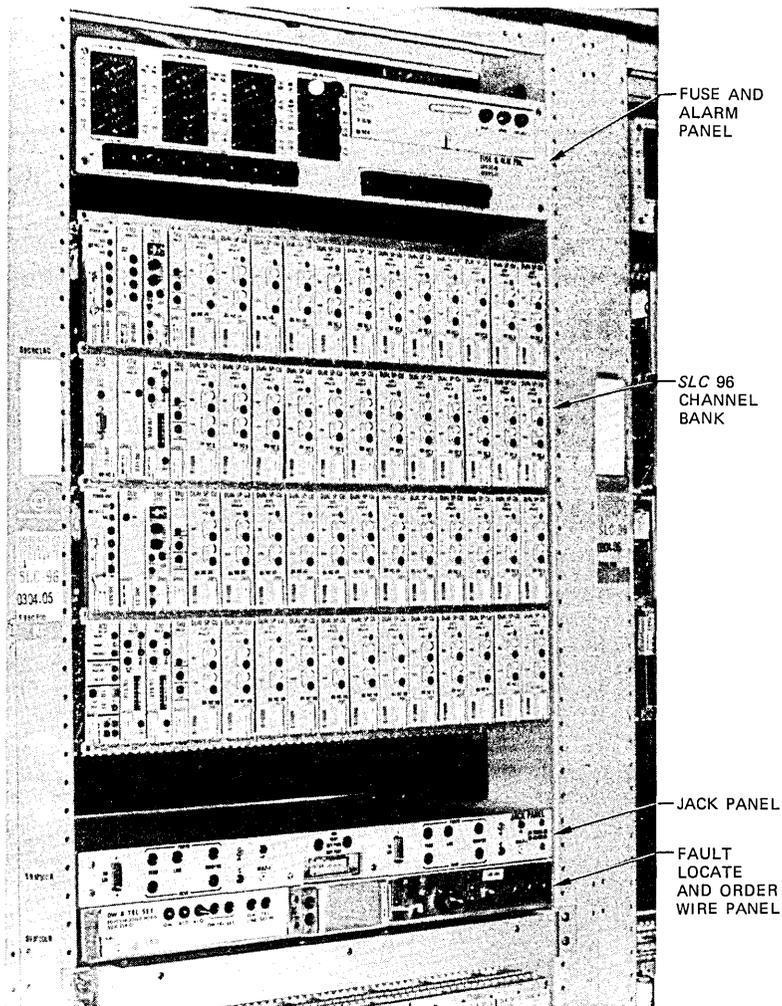
Fig. 1—*SLC 96* carrier—central office channel bank.
