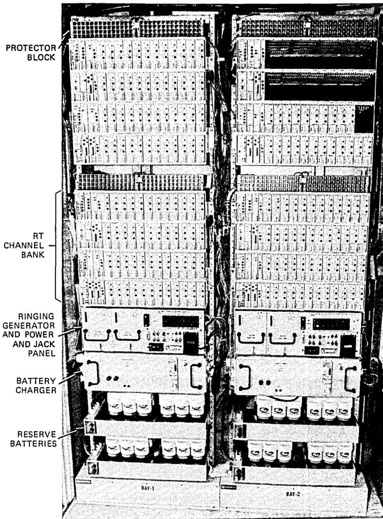
Fig. 7—Remote terminal equipment mounted on a 7-foot bay.
