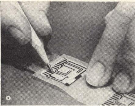
shows the user transferring conductor pattern to wafer by rubbing with pencil point. In photo 3 (upper right), conductor pattern has been etched and resistor pattern applied to wafer. User is now etching resistor in beaker of solution mixed from two bottles in background. Photo 4 (lower right) shows complete amplifier circuit with externally-mounted components.
