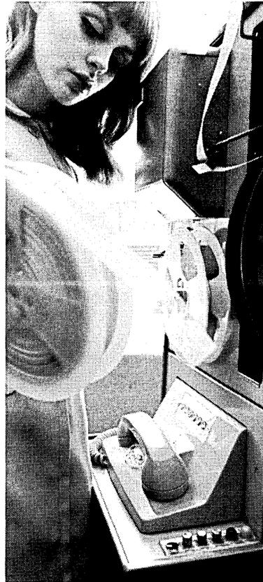
The transmission takes only a few minutes, at most. Some *Telespeed* sets automatically check the transmission for errors, and make corrections, at the same time.
