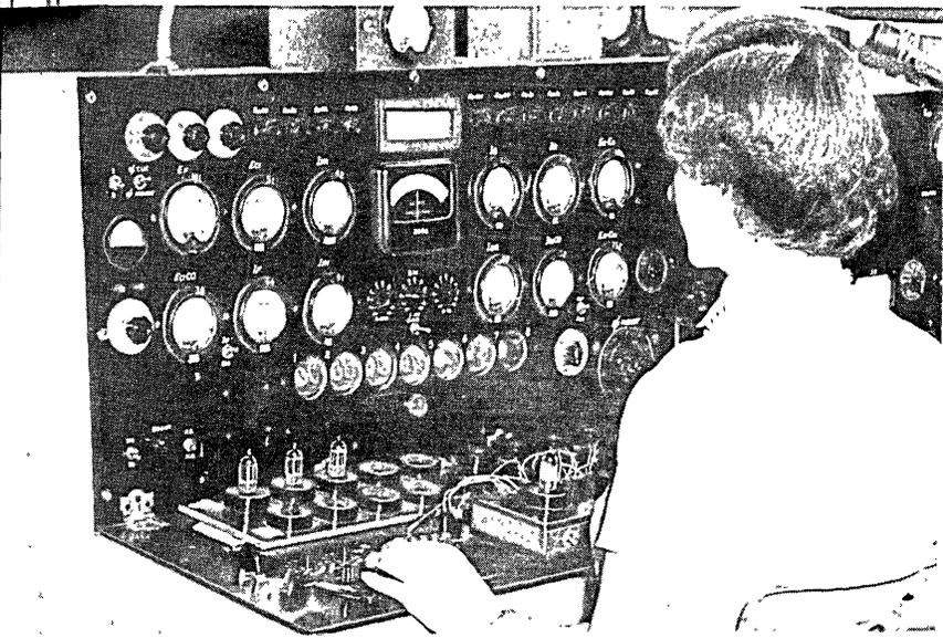
RIGHT: extensive instrumentation is used to test tube electrical qualities that closely affect operation in computer circuits. Zero-bias plate current; cut-off performance; any difference in cut-off between twin-triode sections—these are three of many characteristics checked. ▶
