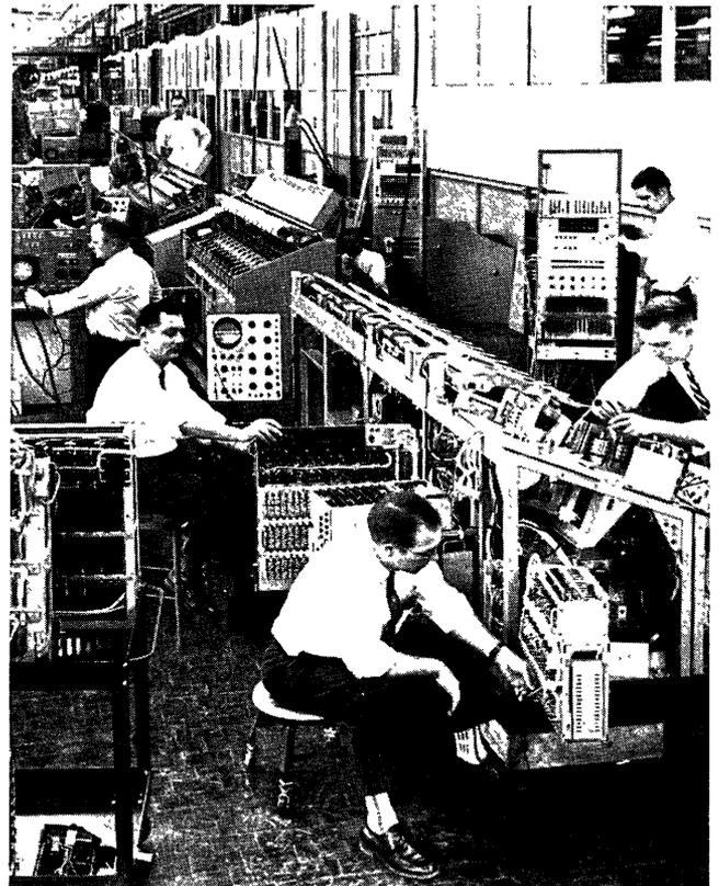
Burroughs Corp. engineers and technicians are shown working on a portion of the production line set up by the company to produce MICR (magnetic ink character recognition) electronic sorter-readers. The \$63,000 machine reads and processes bank documents at speeds up to 26 items a second.
