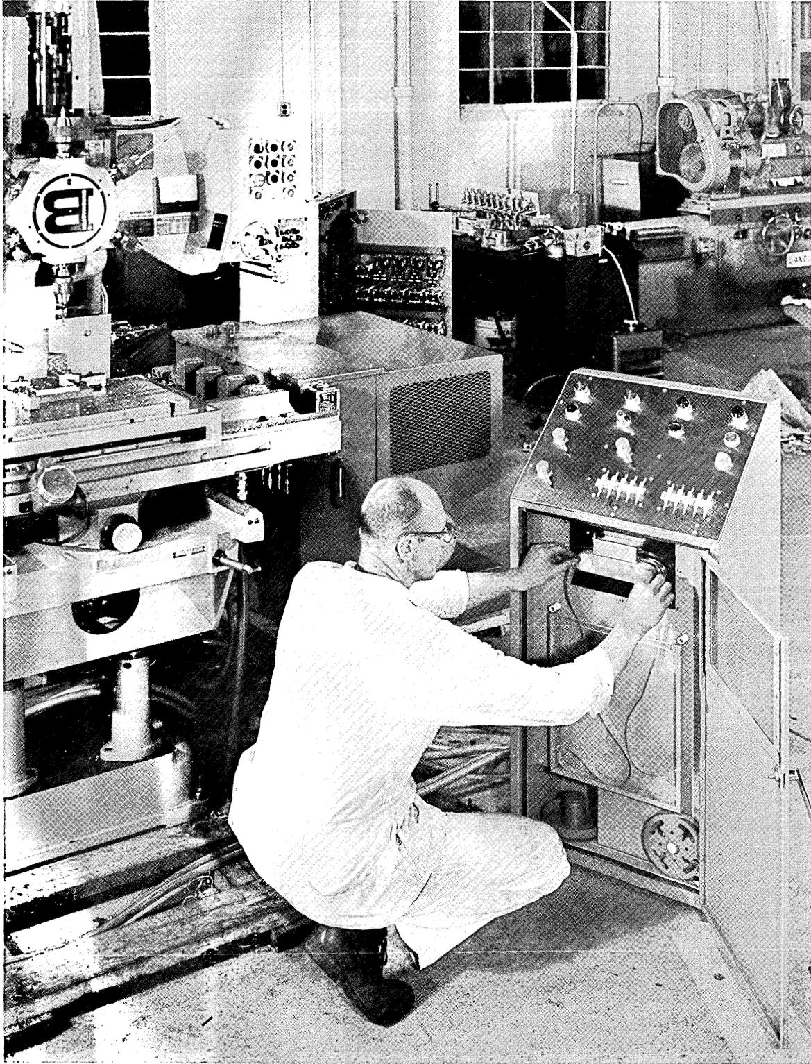
Hydra-Point, a pneumatic-hydraulic system for automating machine tools -- Industrial Division of Moog Servocontrols, Inc., East Aurora, N.Y. An operator inserts punched tape into the console of the Hydra-Point numerical control system. The power supply is shown in the center rear. It was developed as a result of experience in hydraulic control systems for missiles and aviation industry, and its advantages are said to be simplicity of design, speed of operation, accuracy, and low cost.
