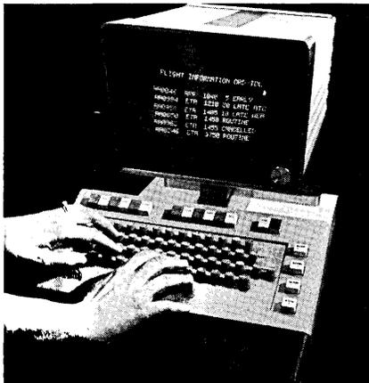
— Messages, queries and replies to and from the computer are composed on the alphanumeric keyboard and confirmed on the CRT screen.
