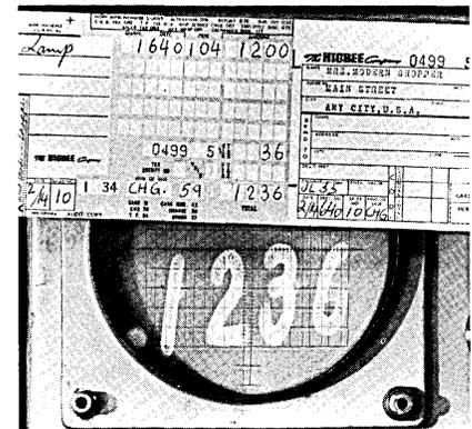
— The total from a handwritten sales check, \$12.36, is displayed on an oscilloscope after the four numbers have been scanned by an experimental IBM optical reader.
