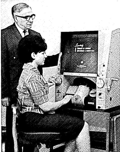
— New device can turn out copies of microfilmed documents in less than three seconds.
