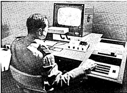
ground cards, a PARD operator punches four coded buttons, shown at right in the picture. Within six seconds the correct card is located and popped up. The operator removes the card and inserts it in the Microteleviser (to operator's left in the picture) which enlarges the microfilm image up to 250 times. This image appears on a television screen in front of the operator, as well as on any number of large and small screen television displays.
