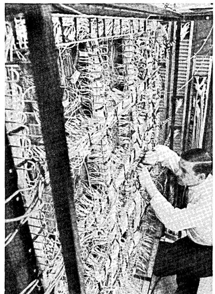
— This electronic arithmetic unit is part of a "super computer" now being built at IBM's Poughkeepsie (N.Y.) plant.
