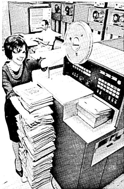
— SSA supervisor Sharon Trieber balances four-foot stack of earnings reports that the optical page reader has condensed onto a single reel of magnetic tape
