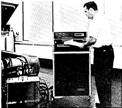
— Service technician runs sequence of automobile engine and electrical systems tests on Allen 1280 automotive computer.
