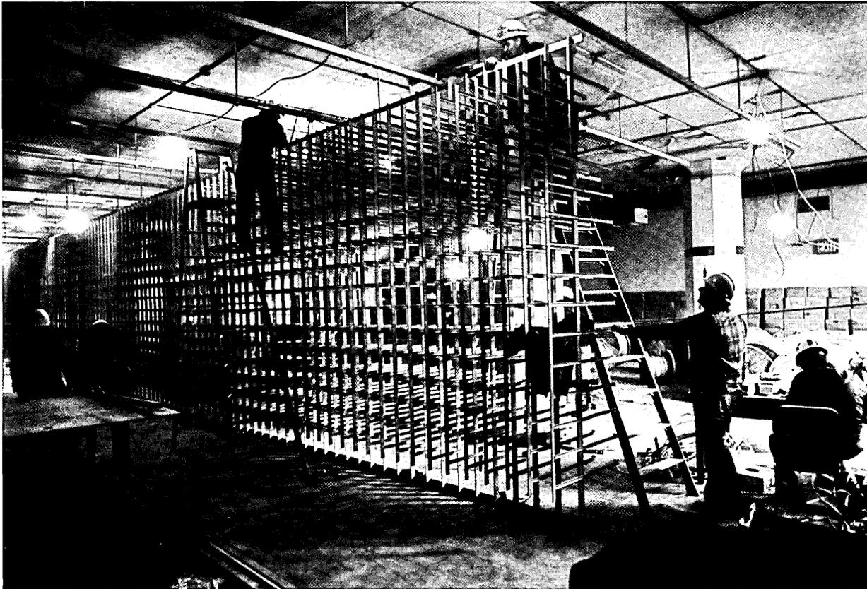
Installers began assembling a new main distributing frame in the Second Avenue building just two days after the fire was quelled. Two days later, it was completely in place.
