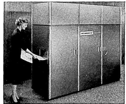
STROMBERG-CARLSON Co., Rochester 3, N. Y., has announced a new high-speed electronic printer, the S-C 5000, that will print the output of electronic computers at 4,680 lines (about 65') per minute, and can be used in both the on-line method of receiving electronic data direct from the computer, and the off-line method of receiving data from magnetic tape.
