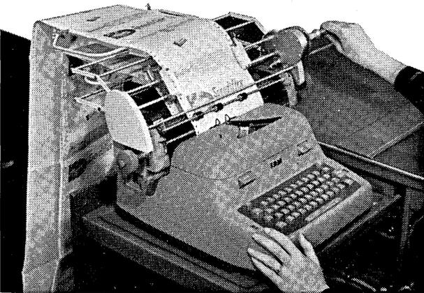
Get continuous production from typewriters or bookkeeping machines. Moore Flexible Formliner permits use of continuous forms in typing; Vertical Spacer skips forms past non-write areas.
