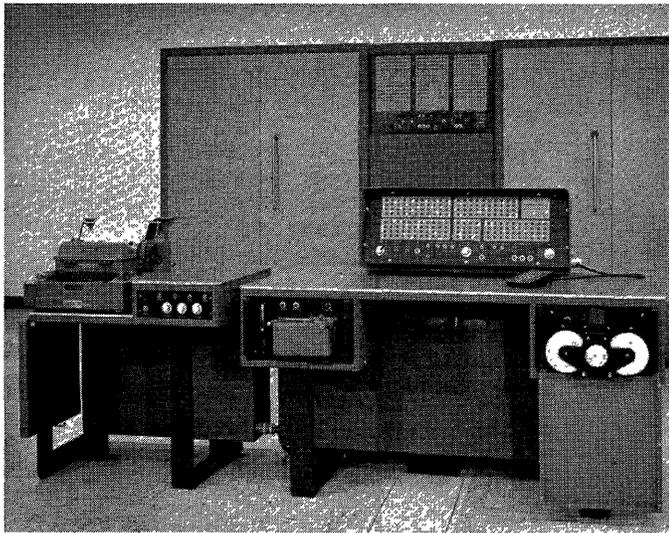
Fig. 6. ElectroData digital computer
