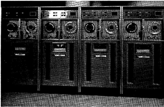
Fig. 6 A group of UNIVAC tape units.
