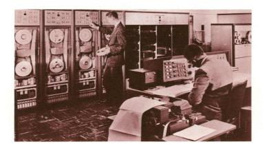
Ampex Computer Tape Handlers shown here used in National Cash Register's NCR-304 Computer system as installed in Macy's, the world's biggest, busiest store. These same instruments are used in Philco's Transac S-2000 Computer, and Control Data Corporation's Model 1604.
