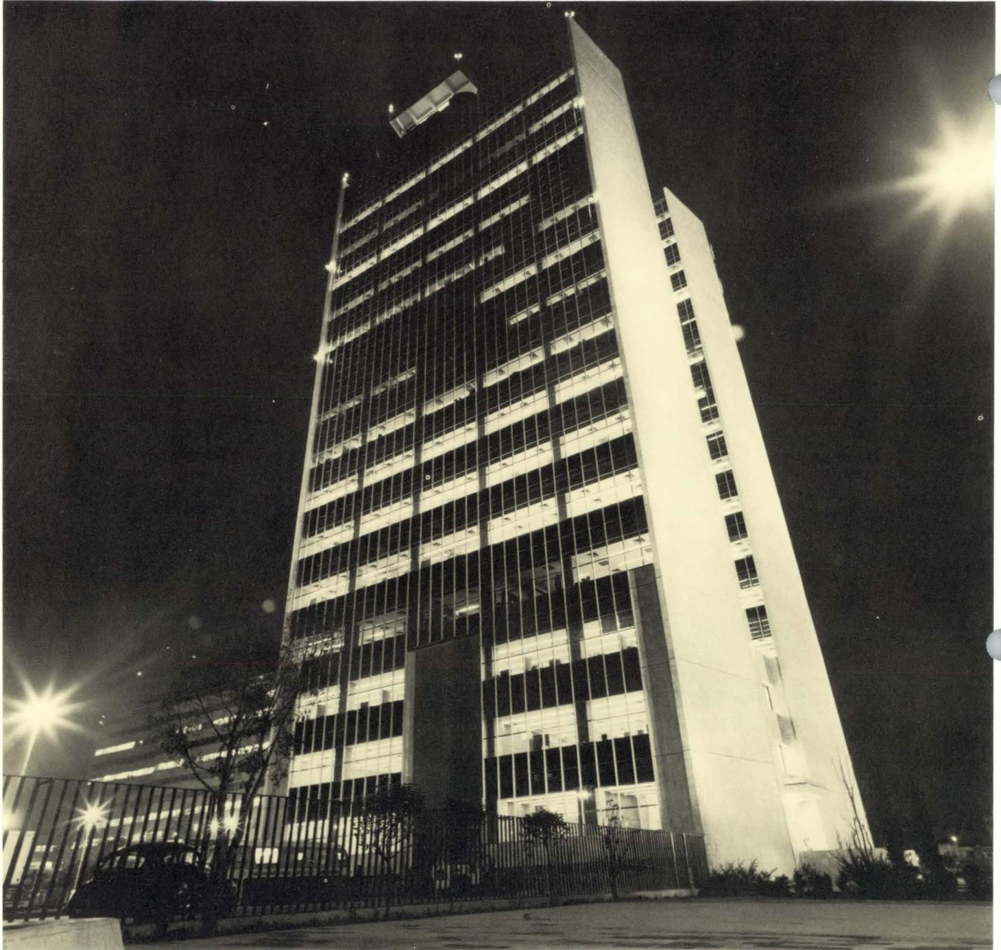
*Fifteen-story Communications Tower rushed to completion by Mexican Ministry of Communications housed recording, switching, monitoring and microwave transmission gear. Antenna dishes on the roof linked the tower with cameras at the various venues around the city and relay stations to the U.S. and overseas satellites.*
