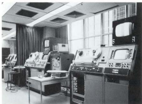
Overall view showing three of EBU's six VR-2000 recorders.
