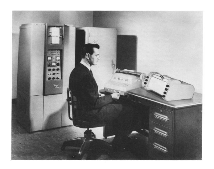
Left to right are pictured the G-15 Computer, the DA-1 Accessory, the input-output typewriter supplied with the computer, and the PA-3 x-y Plotter used for graphical output from the DA-1.
