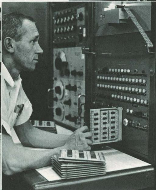
Quality control is assured by modern inspection equipment which automatically tests third-generation, monolithic circuit boards.
