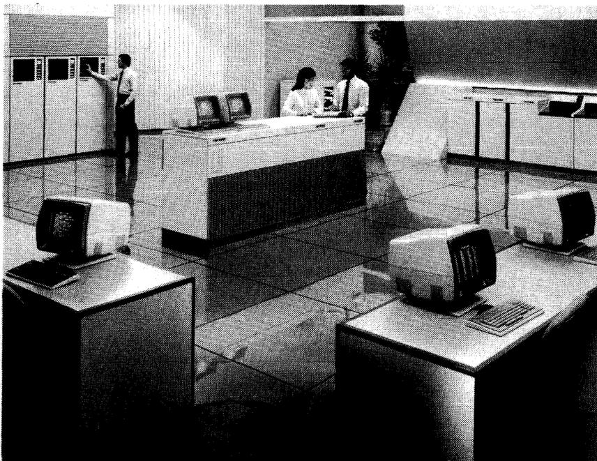
*Burroughs' A 9 Model D and Model F are general-purpose mainframes with a main memory range from 6 to 24 megabytes. The A 9 systems feature a full range of compilers, data management facilities, and applications generation systems. Model D is field upgradable to the Model F.*
