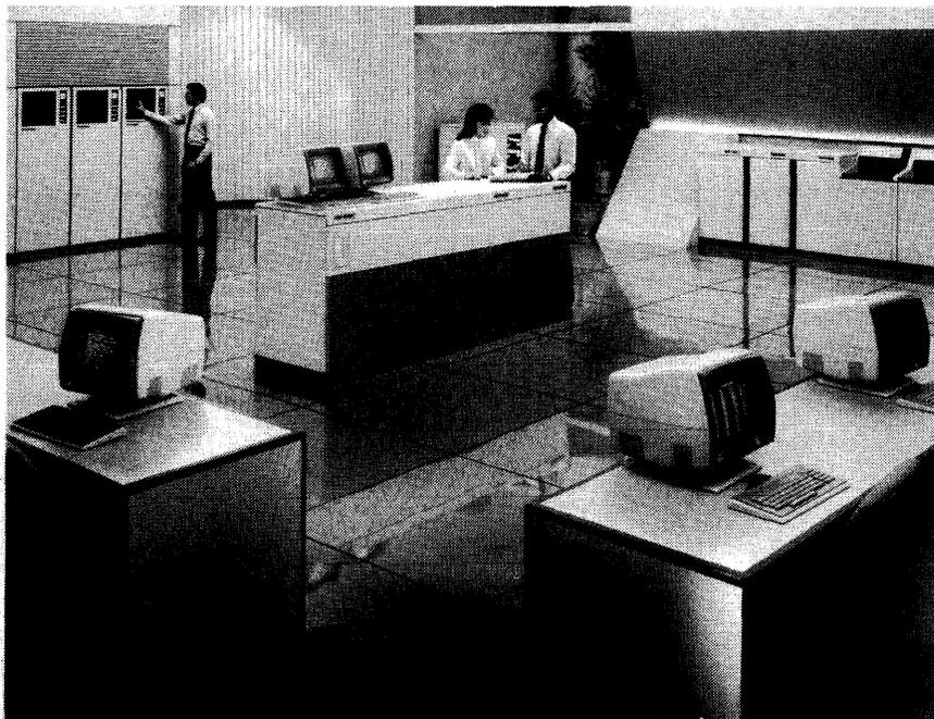
*The Unisys A 9 System is a general-purpose mainframe with a main memory range from 12 to 24 megabytes. The system includes two I/O cabinets with up to 40 Data Link Processors.*
