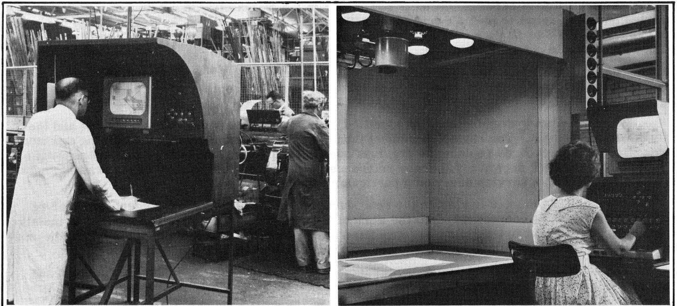
CLOSED-CIRCUIT TELEVISION MASTER STATION (at left) provides visual production drawing information to shop personnel at plant floor CLOSED-CIRCUIT TELEVISION MONITORS (at right).
