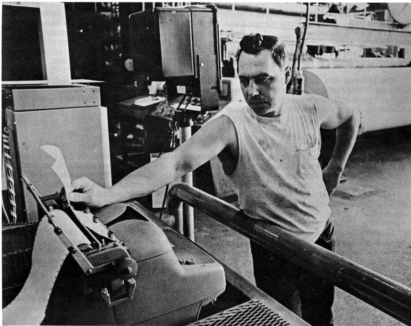
REPORTS ON PROCESS VARIABLES AND INSTRUCTIONS FOR ADJUSTING THE PAPER MACHINE ARE ISSUED BY COMPUTER AND PRINTED OUT.
