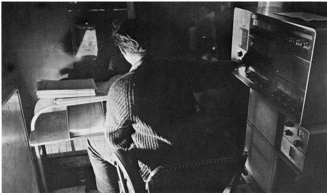
A QUALITY CONTROL OBSERVER FEEDING INFORMATION BASED ON VISUAL INFORMATION INTO AN ELLIOTT 803 COMPUTER SYSTEM. THIS INFORMATION DEALS WITH SURFACE QUALITY OF THE SLAB AS IT IS BEING ROLLED.
