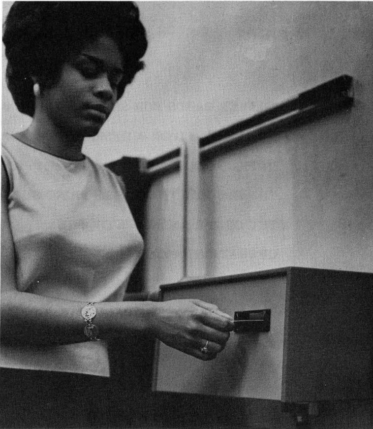
TIME RECORDING EQUIPMENT AT AMERICAN BOSCH IS CONNECTED DIRECTLY TO THE DATA PROCESSING CENTER. EMPLOYEES INSERT PLASTIC CARDS INTO THE IBM 1035 DATA COLLECTION TERMINAL, AND TIME IN AND OUT IS RECORDED ON A PUNCHED CARD AT THE DATA PROCESSING CENTER.
