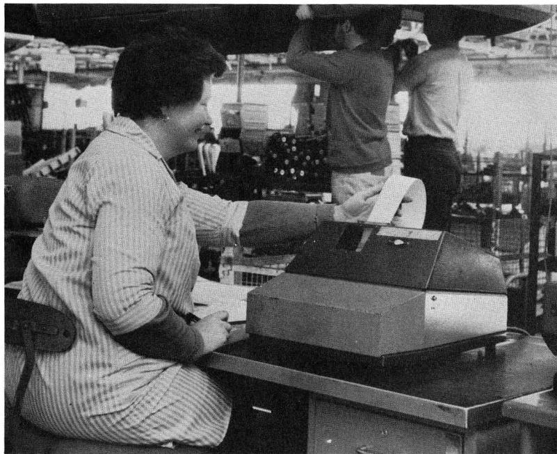
OPERATORS ON THE ASSEMBLY TRACK RECEIVE THE INFORMATION ON I. C. T. PRINTING DEVICES ABOUT ONE-AND-A-HALF HOURS BEFORE ARRIVAL OF THE RELATED CAR BODY.
