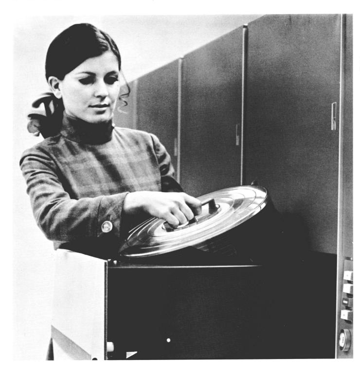
The Control Data 841 Multiple Disk Drive is a large capacity, random access storage device that records and reads information from removable disk packs.
