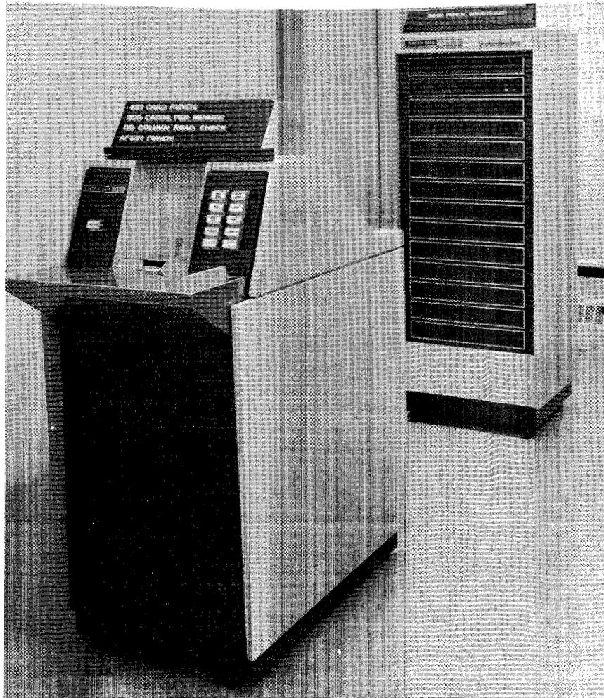
Figure 10-29. Card Punch and Controller.
