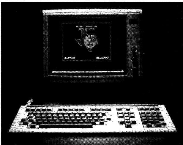
*The Visual 241 is a color graphics terminal that emulates the Digital VT241. The Visual 241 supports Tektronix 4010/4014 and Digital ReGIS graphics protocols, making the unit compatible with a wide variety of graphics software packages. A 13-inch display screen with an 80/132-column display format is standard.*
