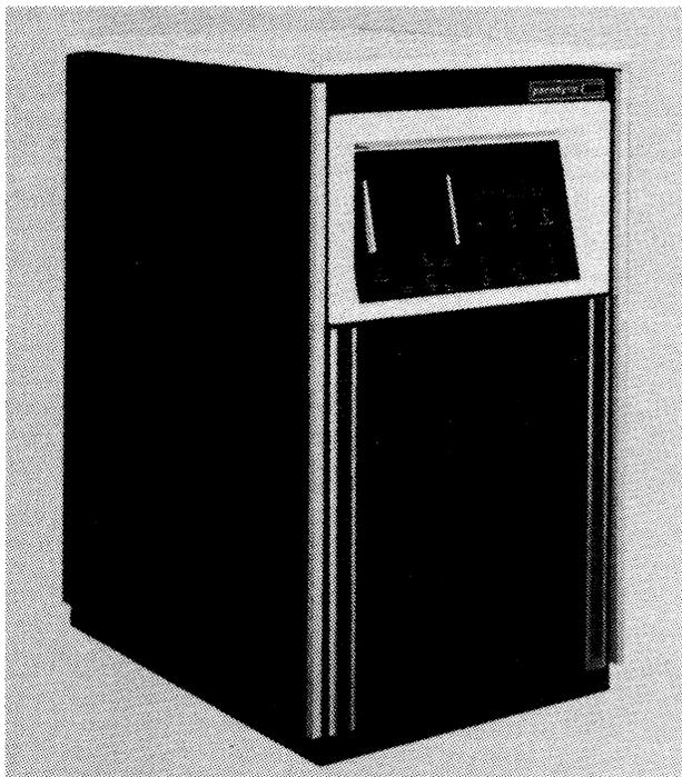
The PIX Remote Control Unit (RCU) can be located locally or remotely to the host computer, and communicates with the host via a PIX Local Control Unit (LCU). Up to 25 peripheral devices/controllers can be physically connected to an RCU. The maximum number of device addresses that can be handled by an RCU is 64.
