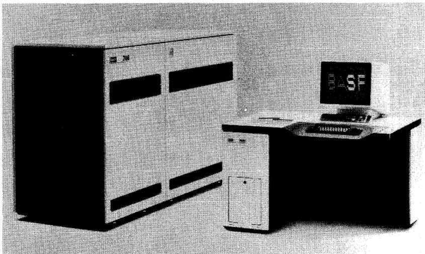
*The BASF 7/68, a plug-compatible substitute for the IBM 4341-2, is based on the Hitachi M240H and can support both IBM and BASF peripherals. BASF reports that tests show the 7/68 about twice as fast as the 4341-2 while taking up less space and generating less heat.*
