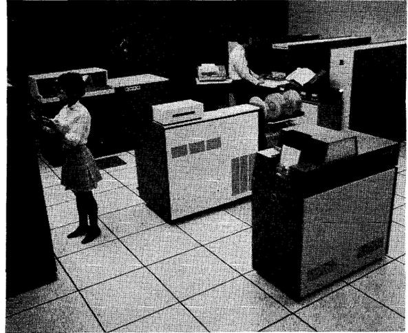
*Multiprogramming of 4 to 10 independent jobs is an everyday way of life for B 3500 installations such as this one. The central processor is at right rear.*
