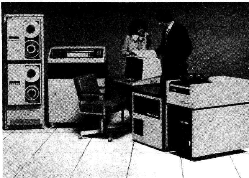
The Cyber 18-20 features a memory size of from 32K to 256K bytes, 9 I/O slots that accept magnetic tape, floppy and hard disks, a card reader/line printer, and micro memory controllers. A typical 18-20 system with 192K bytes of memory, ten terminals, 300 lpm printer, and 100 megabytes of disk storage costs about \$115,000.
