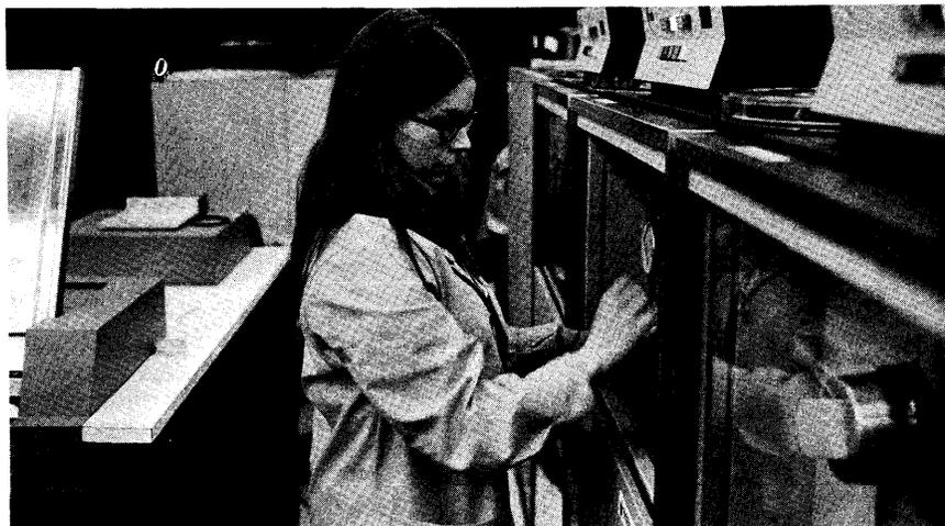
*Phoenix System buyers can elect to use magnetic tape units and disk drives manufactured by either IBM or CalComp. Punched card I/O functions will normally be handled by the familiar IBM 2540 Card Read Punch at left.*
