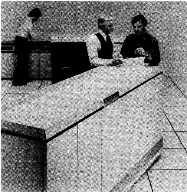
*The Series 68, the top-of-the-line Series 3000, performs at the one-million-instructions-per-second level. The system offers many advantages of a 32-bit machine—a 32-bit data path, a 32-bit memory word, and dual arithmetic logic units—while maintaining full compatibility with existing HP software. The system shown here includes multiple disk units, an additional I/O bay, and HP's laser printer.*
