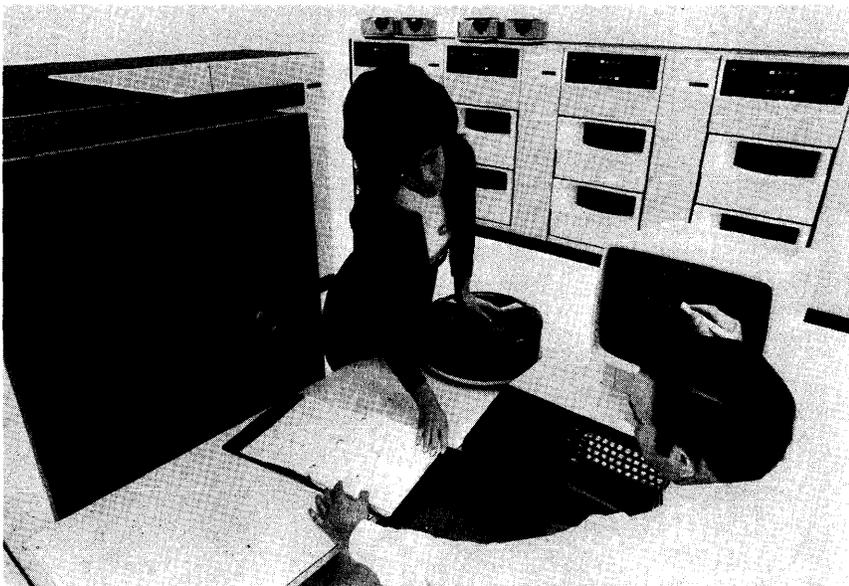
*Enhanced by IBM's February 1973 announcements, the Model 158 Processing Unit now provides up to 4 million bytes of MOS main storage and is available in both uni-processor and dual-processor (MP) configurations. A feature of the Model 158 is its CRT display console with light-pen input. An 8-drive 3330 Disk Storage subsystem is in the background.*
