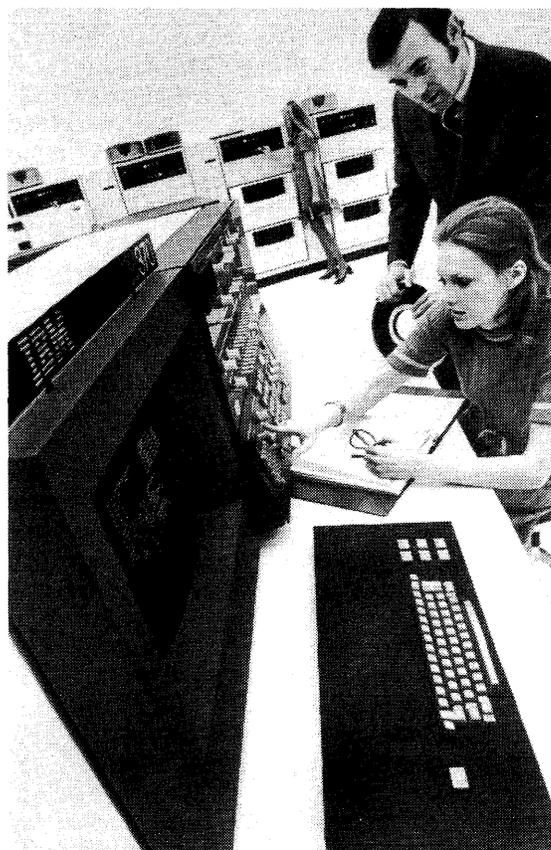
*The largest of IBM's virtual storage computers, the Model 168 and its enhanced successor, the Model 168-3, offer up to 8 million bytes of real MOS main storage. A dual-processor Model 168 MP system can include up to 16 million bytes. The Model 168-3, announced in March 1975, features a 5 to 13 percent increase in instruction execution rates and a new Service Processor that expedites on-line error analysis.*
