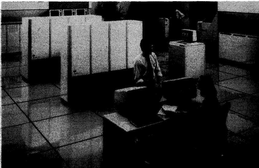
*The Unisys A 15 large-scale system is available in eight models with one to four central processors and a main memory range from 24 to 192 megabytes. The system has one or two I/O subsystems supporting up to 64 Data Link Processors and up to 512 data communications lines.*
