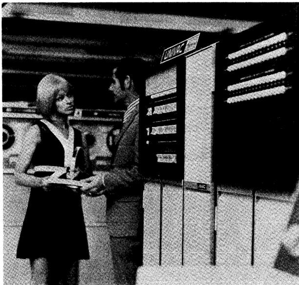
*The Communications/Symbiont Processor (C/SP) is an independently programmed computer designed to control data communications and card and printer I/O operations. It can be used with any of the 1100 Series systems.*
