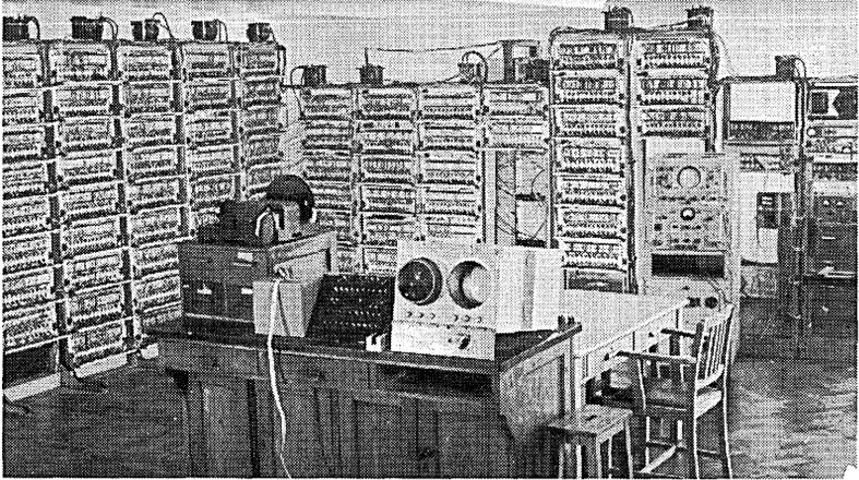
Fig. 7.4 The Manchester University Mark II computer, nicknamed MEG, was 20 times faster than Mark I yet consumed less than half the electrical power. It first worked in May 1954.
