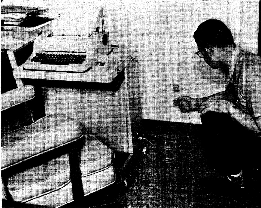
The cabinetry that holds the typewriter and, in its base, all the associated electronics is mounted on casters for mobility and includes a four-way detachable side table that provides a convenient work surface on the left or right side of the console at the user's option.
